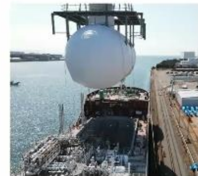
Storage tank installation into the carrier in March 2020
