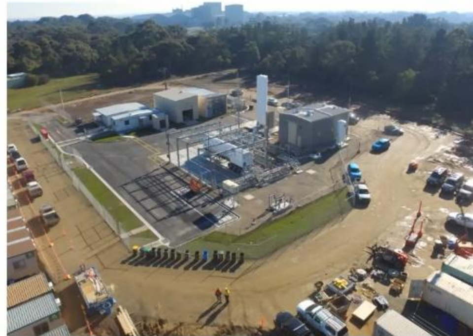
Hydrogen Liquefaction and Storage Plant at Hastings
